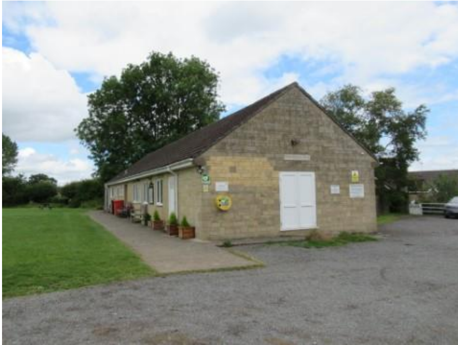
View of the Front Elevation
